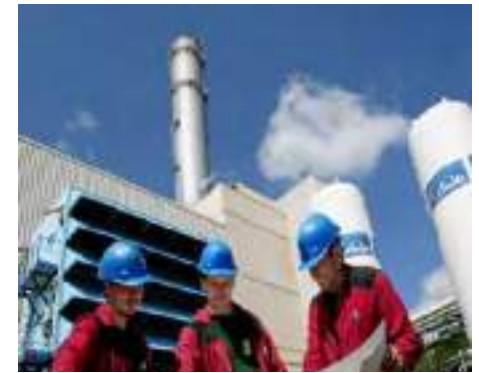
Oxygen plant at the Vresová IGCC power plant in the Czech Republic
